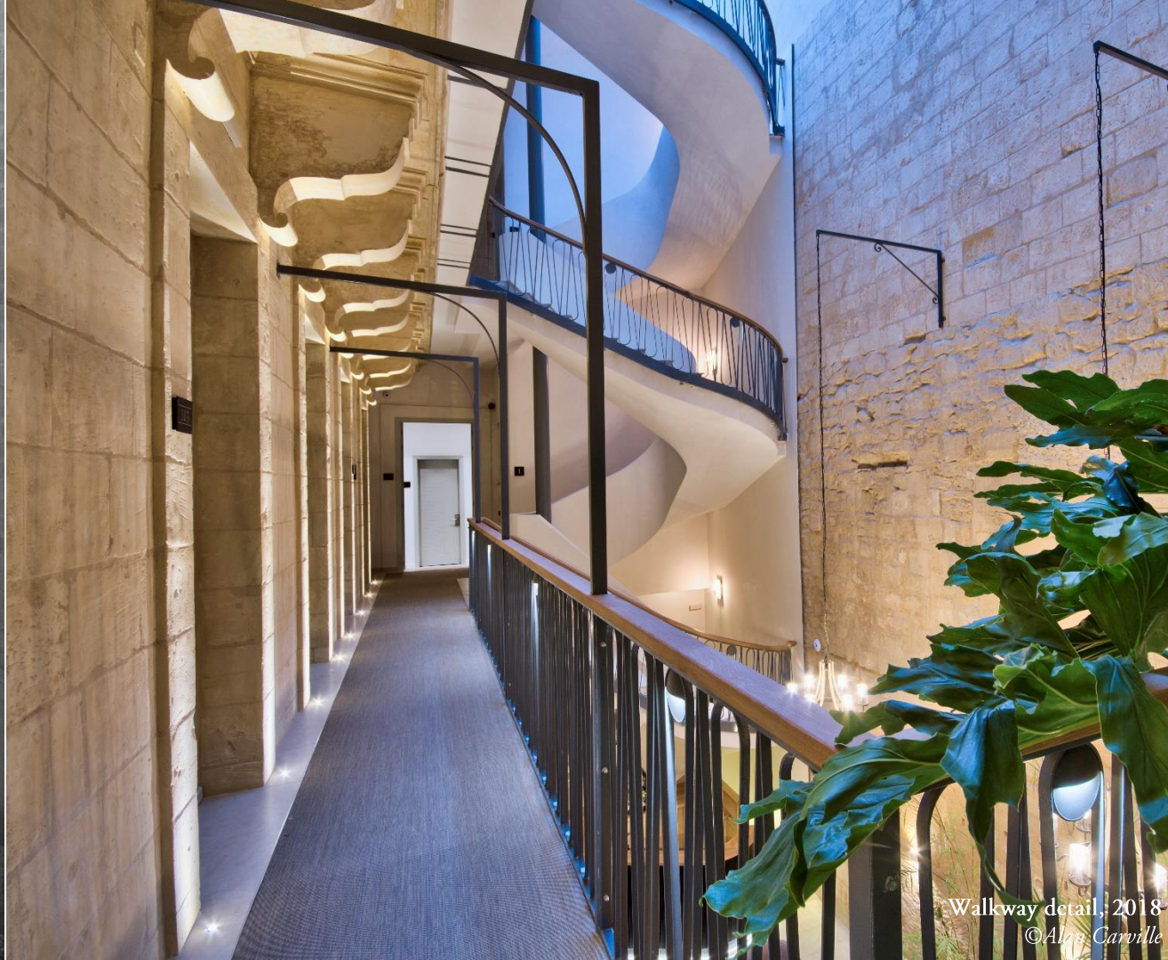
Walkway detail February 2014
